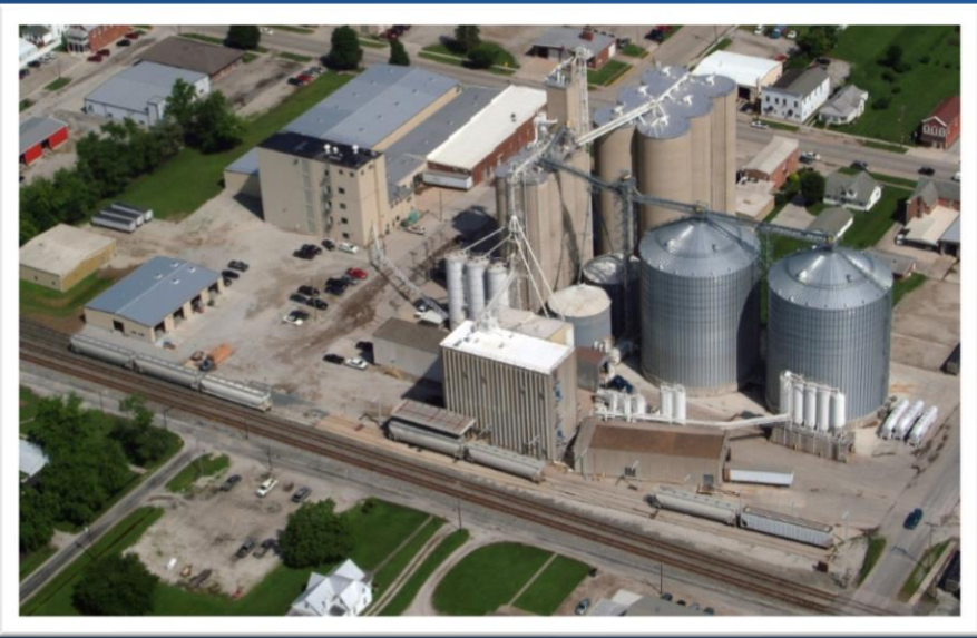
Siemer Milling Company Teutopolis, IL Built in 1979
